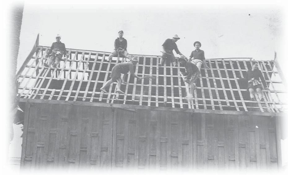
Building a rice granary
